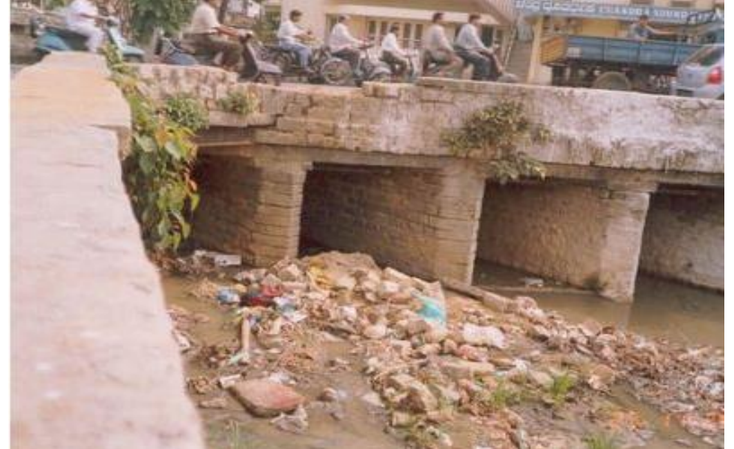
Solid waste dumping-Reduced culvert capacity, inlet block
